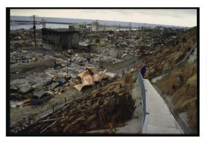
1993 Hokkaido earthquake and tsunami: Aonae, Okushiri Island, looking southeast. Structures in the foreground were damaged by fires fueled by above-ground kerosene and propane tanks following the tsunami. The concrete steps provided a means of escape for some residents following the strong earthquake<sup>2</sup>
