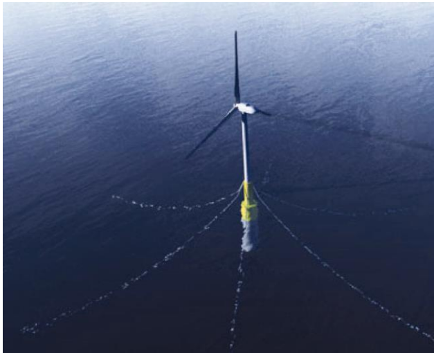
Fig.3. Floating wind turbine 3
